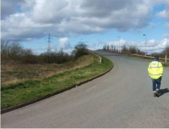
Photo 5: View NW of existing Forrest Way Bridge across the River Mersey
