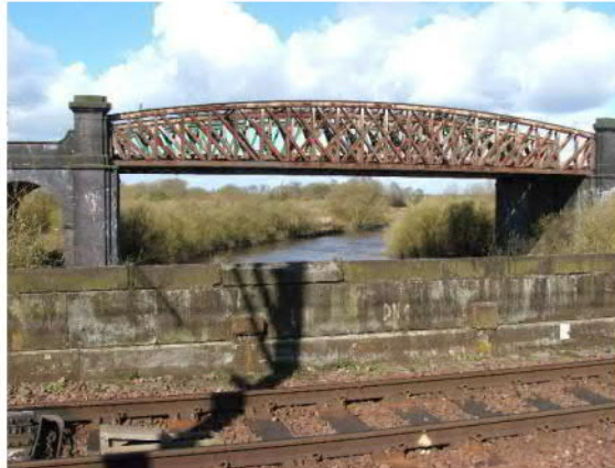
Photo 2: View NW of WCML viaduct across the River Mersey
