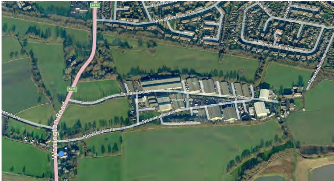
Bird's Eye view of the site from the south
