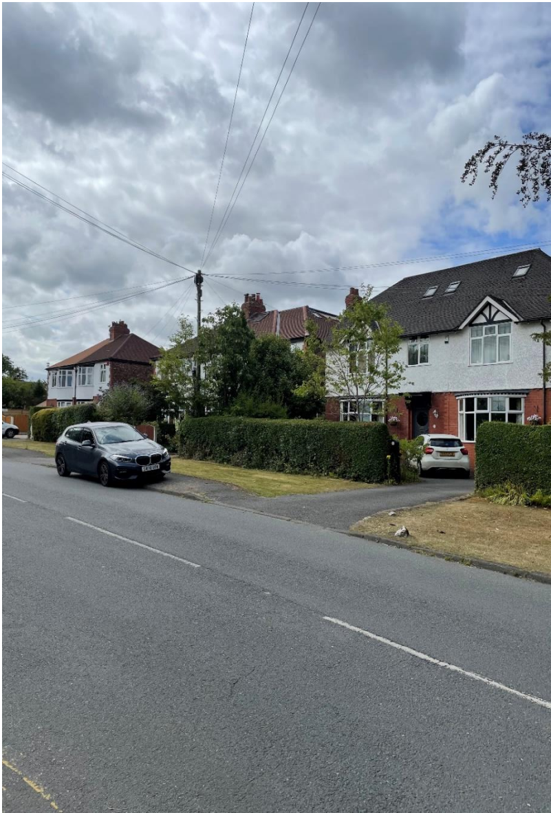
Location 3: Built form along Burford Lane
