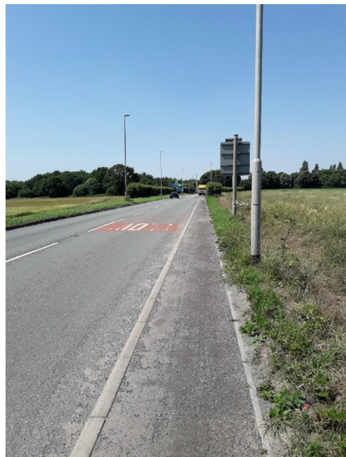
Photo 2.2 – A57 looking west
