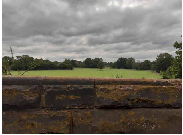
7 View from elevated Stockport Road
