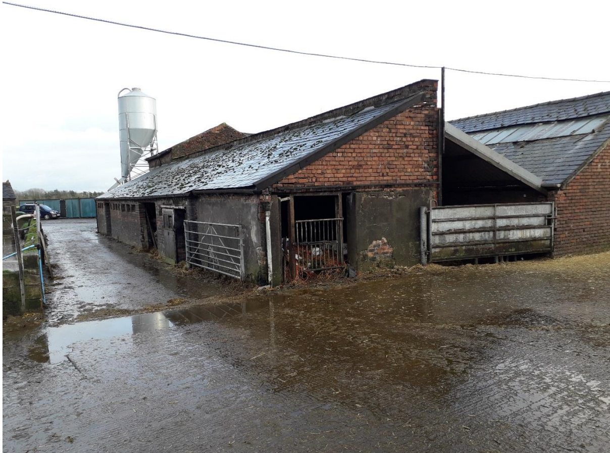
Plate 1 shows 20 th century lean to added to outer wall of former northern range
