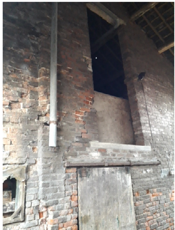
Figure 4: Cracking adjacent to existing openings
