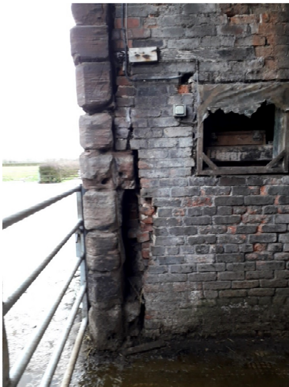
Figure 3: Vertical cracking and separation to rear of entry arch
