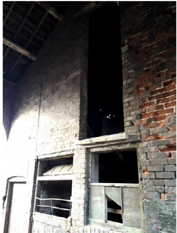
Figure 2: Extensive loss of masonry face to entrance
