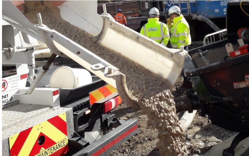
Figure 12: Concrete mix with high cement replacement.
