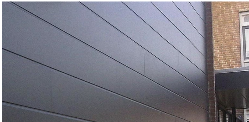
Figure 15: Example of Rockpanel with Rockwool insulation.
