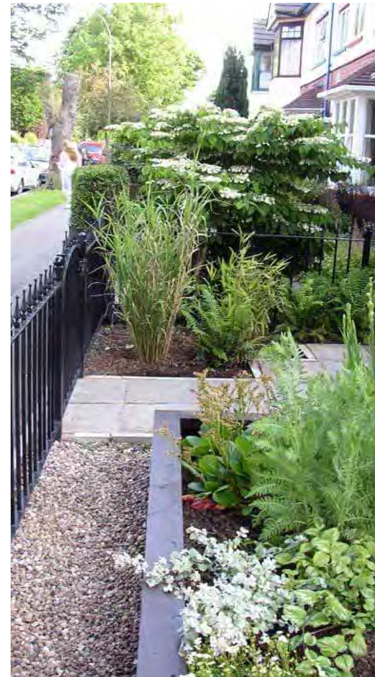
Small scale SuDs such as rain gardens can be a means of mitigating runoff and improving the quality of the street scene
