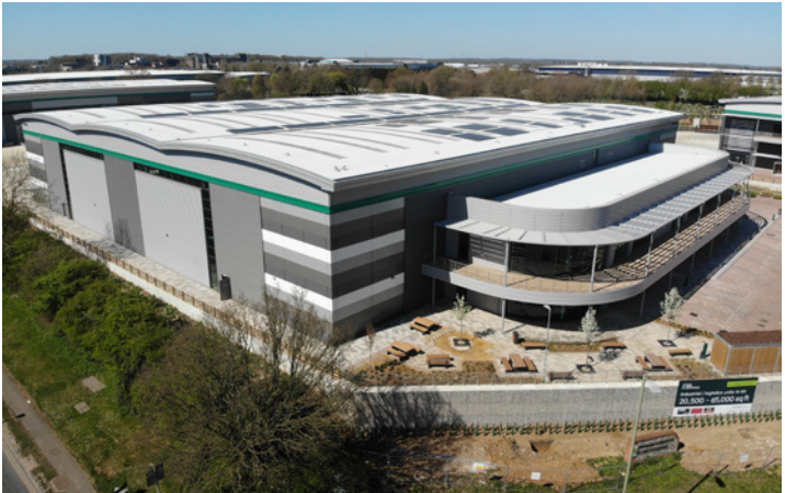
Fig. 47 - Example of B8 industrial unit
