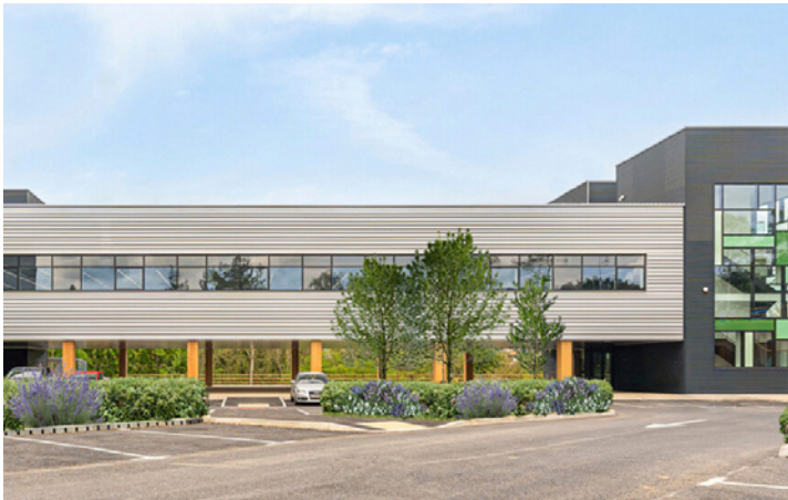
Fig. 184 - Offices overlooking car park
