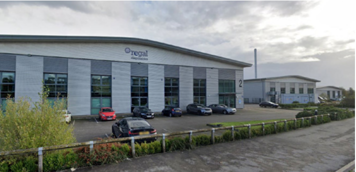
Fig. 5 - Gorsey Point - Small scale industrial units at Bennett's Lane
