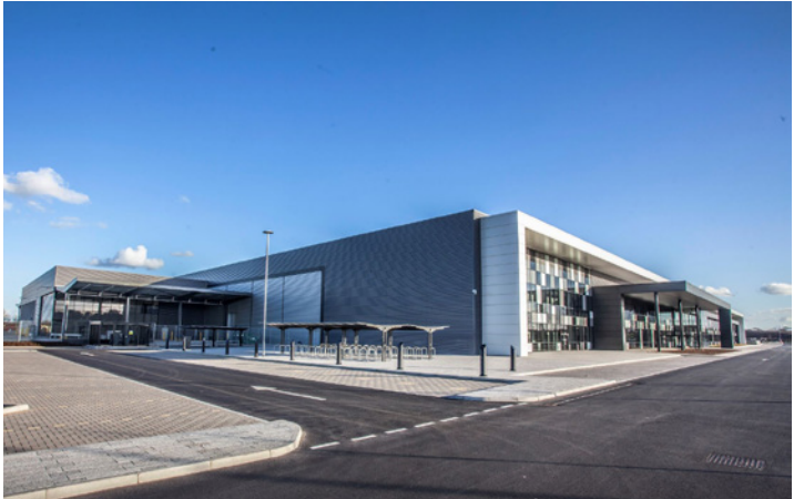
Fig. 46 - Example of B2 industrial unit
