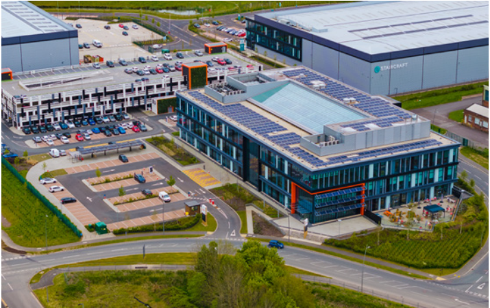
Fig. 44 - B2 general industrial and office unit
