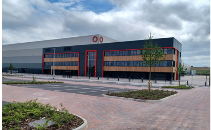
Fig. 43 - Building with offices protruding
