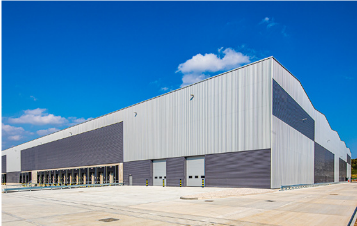
Fig. 49 - Example of B8 industrial units
