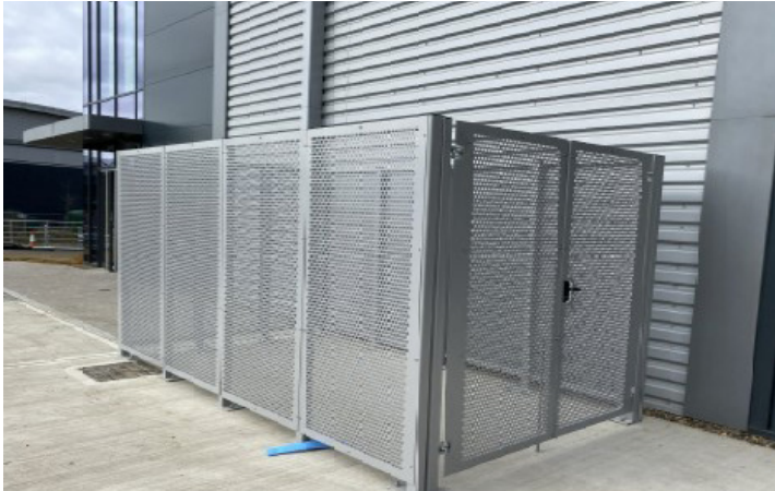
Fig. 77 - Bin enclosure in service yard
