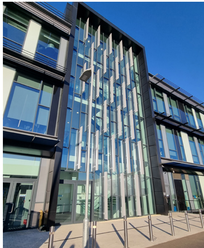
Fig. 73 - External view of double height reception space
