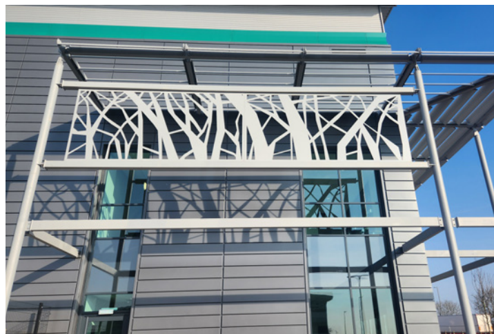
Fig. 176 - External solar shading to mitigate heat gain
