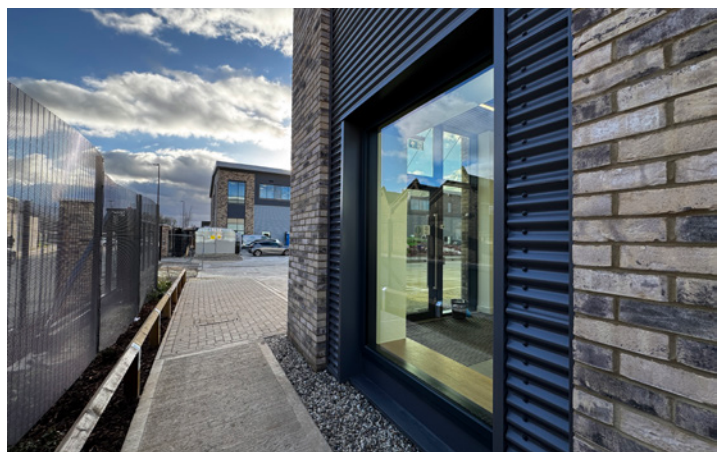
Fig. 191 - Carefully placed windows ensuring surveillance
