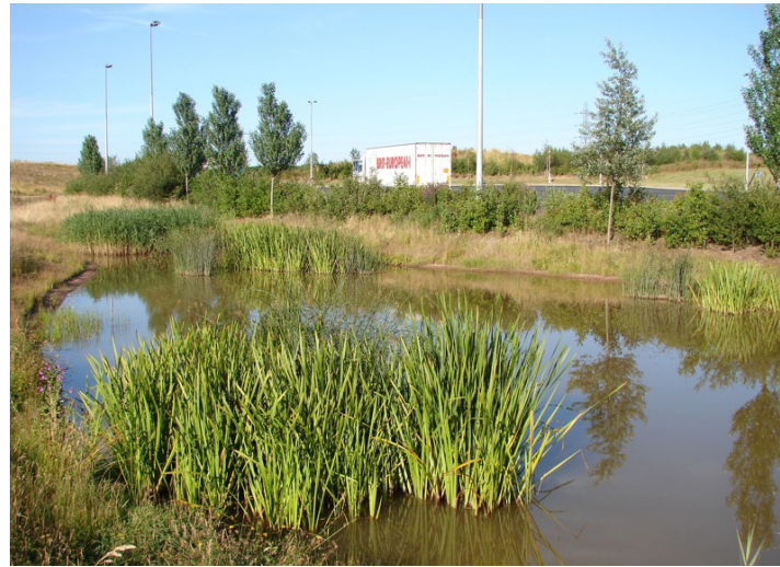
Fig. 154 - Example primary SuDS feature - Pond
