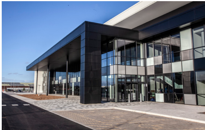
Fig. 67 - Distinctive building entrances
