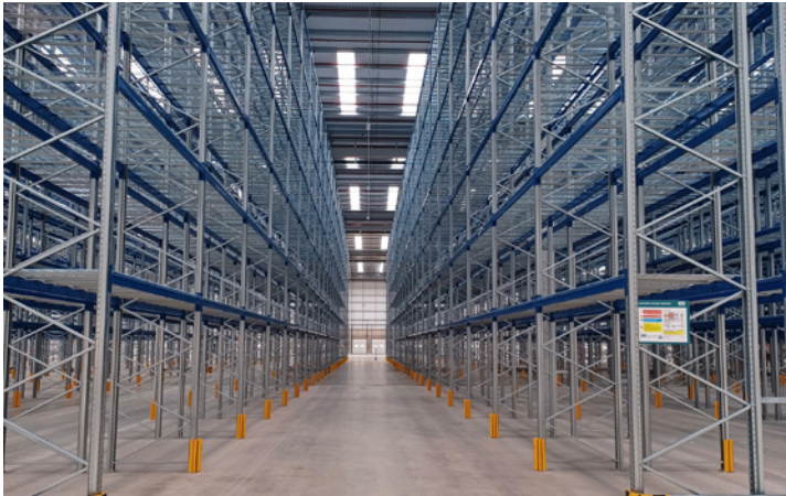
Fig. 50 - Racking inside a B8 unit. Large volumes of space needed for storage means taller building heights.
