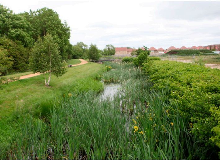
Fig. 149 - Amenity spaces integrated with SuDS conveyance
