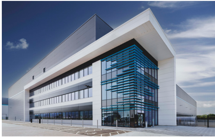
Fig. 34 - Example of B8 industrial unit
