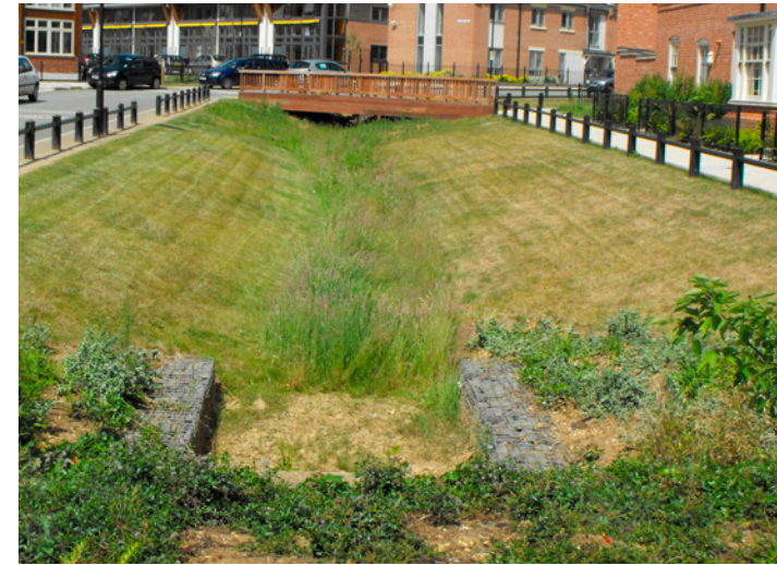
Fig. 155 - Example secondary SuDS infrastructure - Swale
