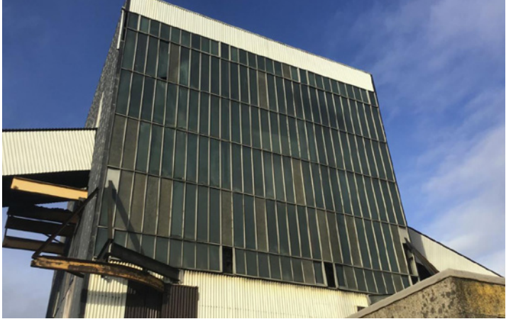
Fig. 58 - Fine grain grid facade
