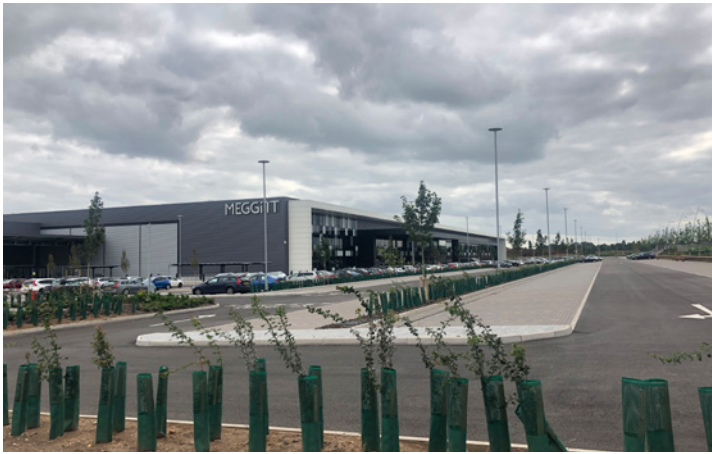
Fig. 31 - Example of B2 industrial unit
