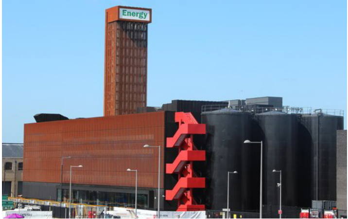
Fig. 61 - Olympic Energy Centre, London
