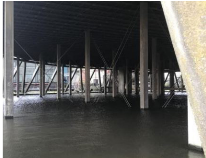
Fig. 14 - Filled cooling tower pond
