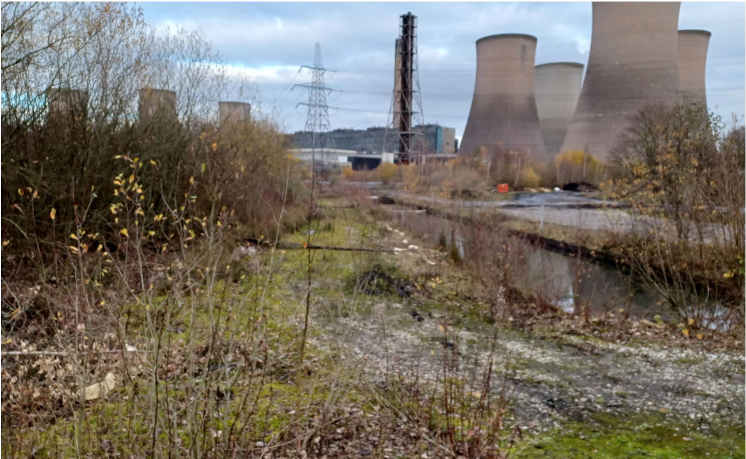
Fig. 29 - View of existing phase 1 employment area looking from the south - Dec 2022
