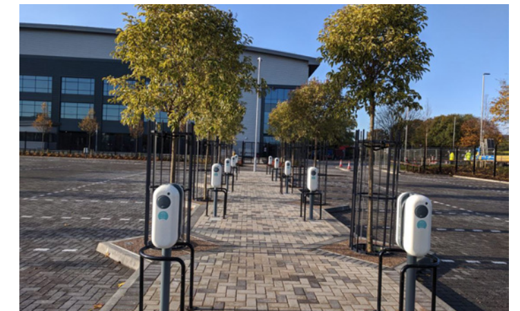
Fig. 108 - Electric vehicle charging points
