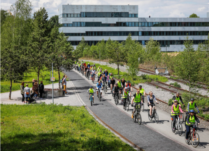
Fig. 124 - Footway / cycleways following historic railway route
